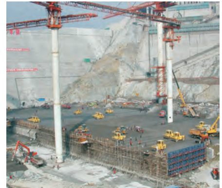
construction of a dam
